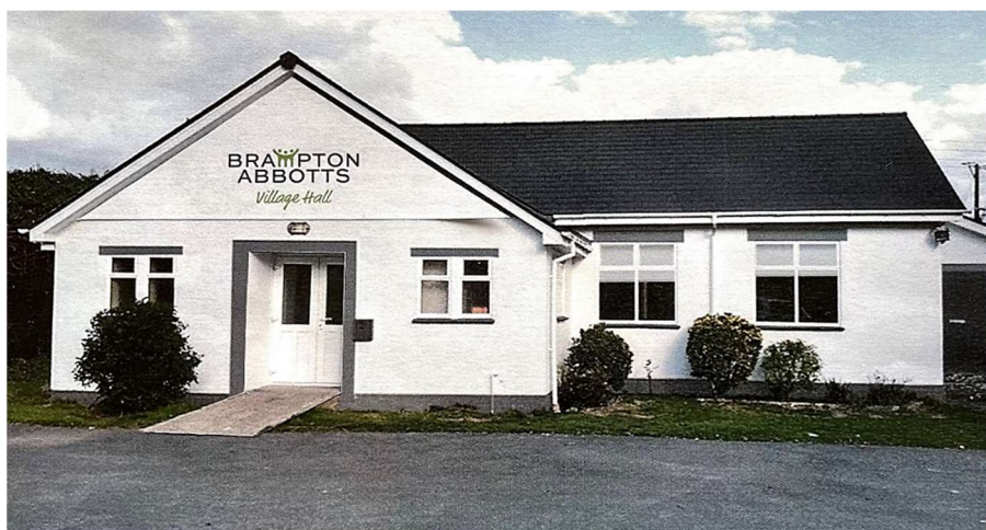
Visual of Hall with branding, painted window lintels, surround to the entrance and the brick work under the damp proof course.
